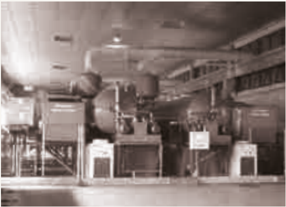
Autoclave treatment station - Moulton production site (14)
